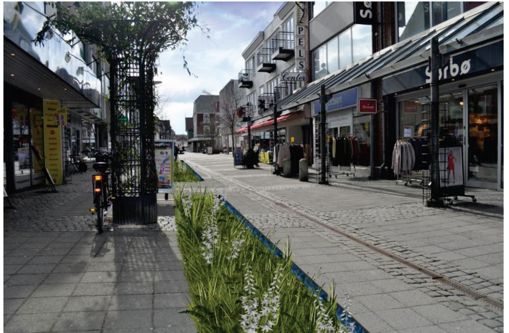
Figure 25. Subsurface storage in Sandnes city with a green surface inlet (without storage volume)
