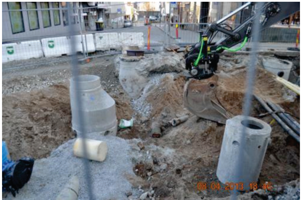
Figure 7. Construction site in study area and infiltration measurements
