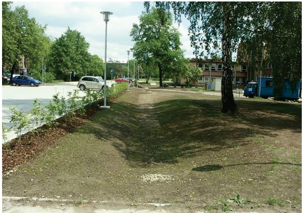
Figure 18. Swale just finished
