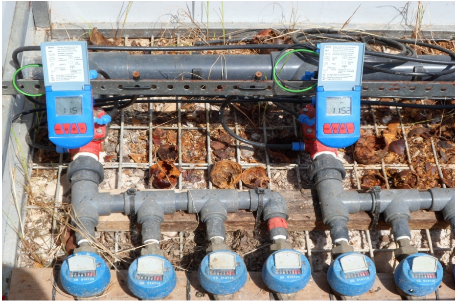
Figure 16. Installation of Programming units and Flow meters.
