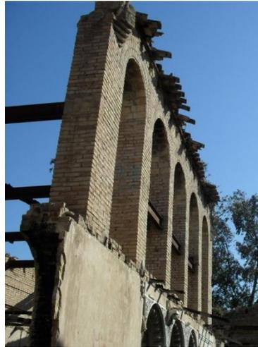
*Fig.74 - Muro portante central (2014)- Fuente propia*
