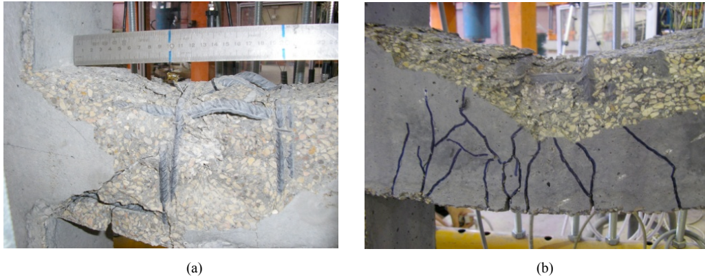
Fig. 7. Spalling of concrete cover: (a) Non-confined column ( \epsilon_s \leq 1\% ) (H60-10.5-C0-2-45) (b) confined column (H90-10.5-C3-2-45)
