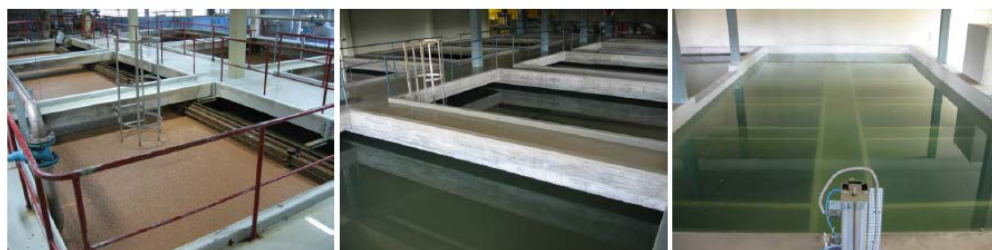
Figure 5 Pictures from the flotation step (left), sedimentation (middle) and filtration (right)
