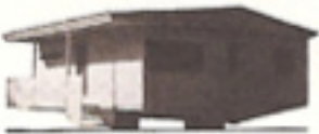
With its narrow foundations, heavily cantilevered form and plywood skin, "Plas-2-Point" house is reminiscent of modern aircraft. Sixteen tons for cold climate would weigh 2 to 4 tons.
