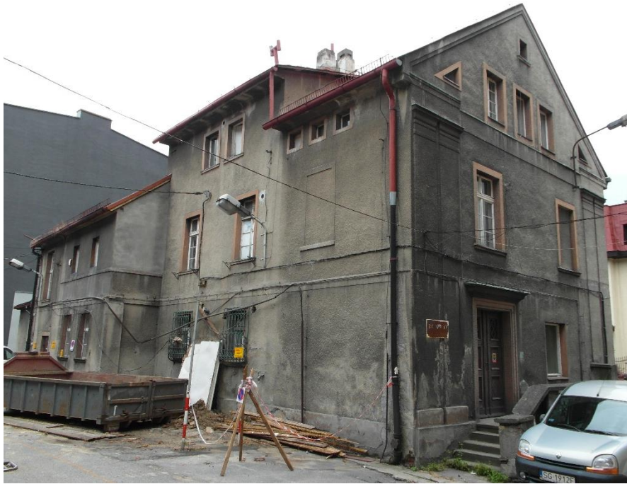
Facade North West
