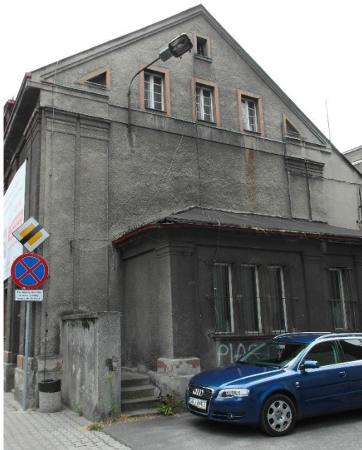
Facade North East
