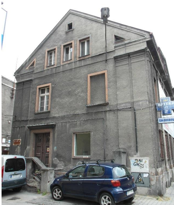
Facade South West
