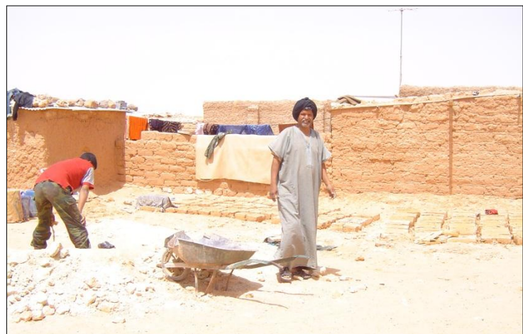
Picture 36. Men at work, mud bricks process construction.
