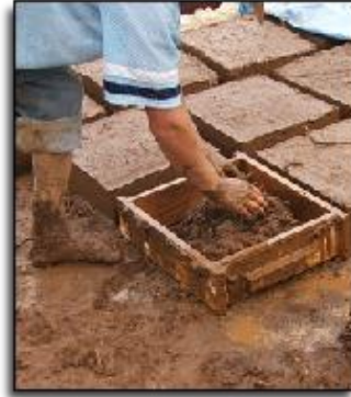
Picture 41. Filling the mold
