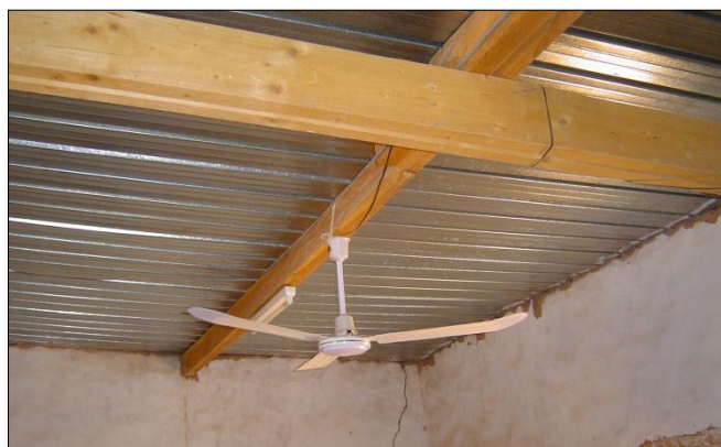
Picture 33. Roof: wood beams and zinc plates.
