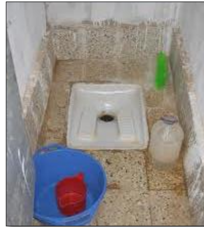
Picture 30 and 31. Toilet (Latrine)
