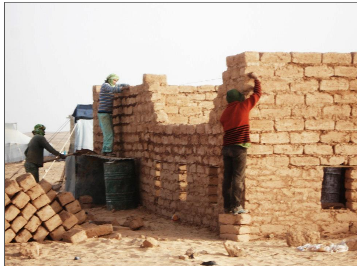
Picture 38. Leveling bricks.
