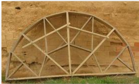
Picture 47. Wooden formwork
