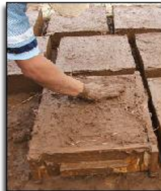
Picture 42. Filling the mold. Pushing mixture
