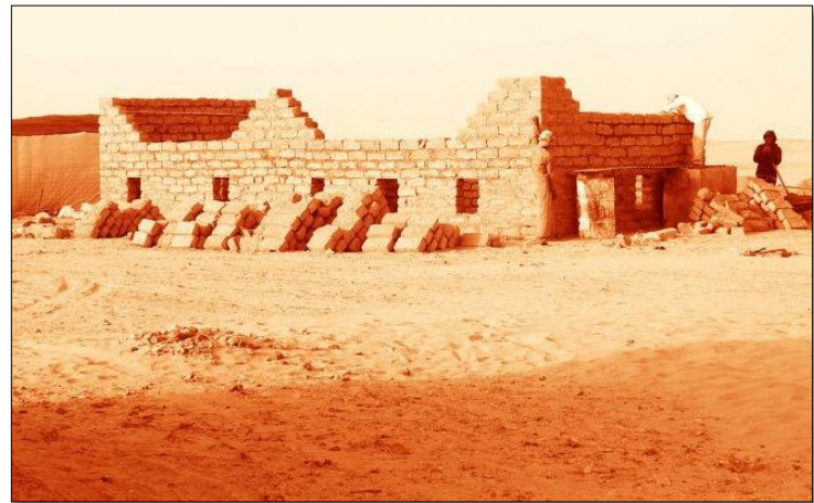
Picture 35. Small windows placed near ground level.
