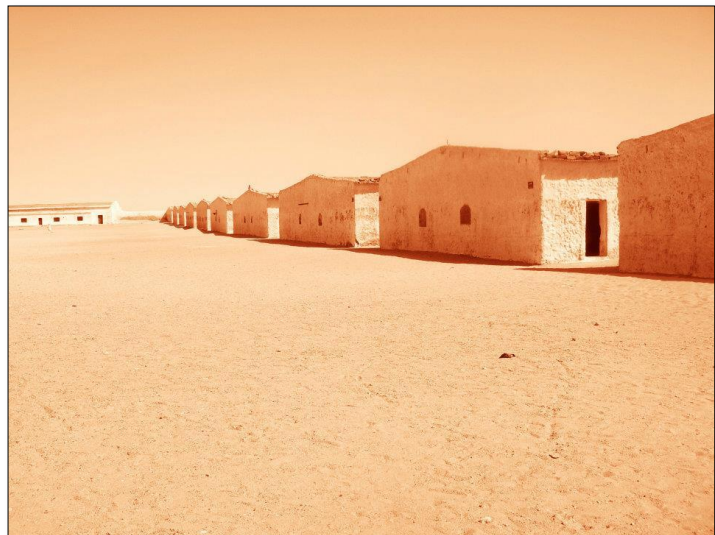
Picture 18. Classrooms 9 th of June Secondary School
