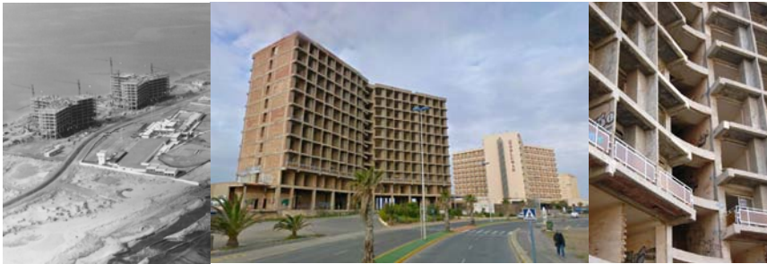
Figure 5: Construction (about 1970) and abandonment a part of Casino Dos Mares. Origin: Archive VECOS promoter and photo authors.
