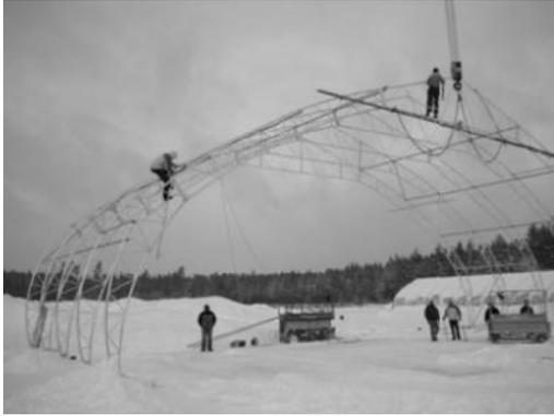
Figure 5a. Greenhouse construction.
