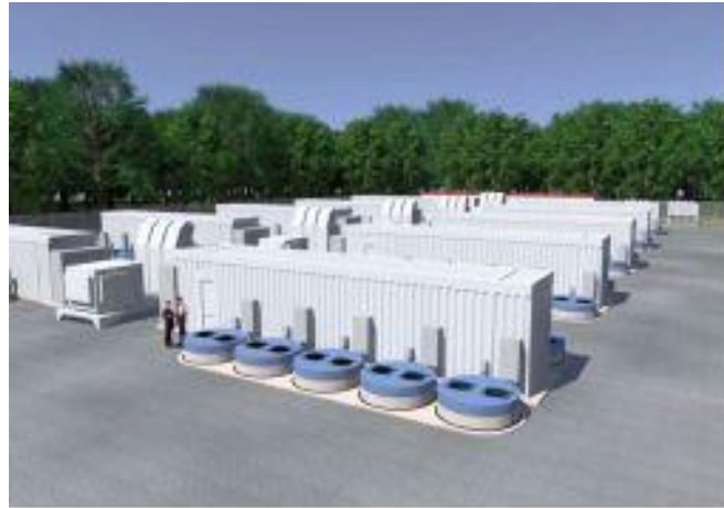
Ilustración 27.- 20 MW, 15-min flywheel frequency refulation plant.
