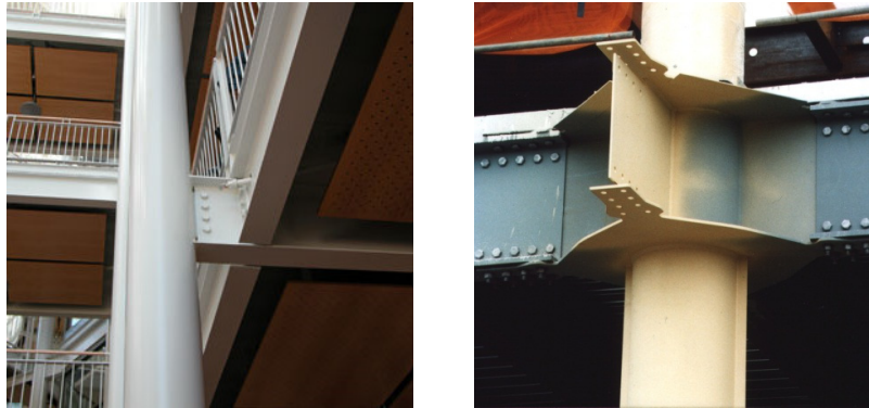
Figure 1.1. a) Shear connection in Transit Terminal in Wisconsin, EEUU [1] b) Seismic connection in Auckland airport, New Zealand [2]
