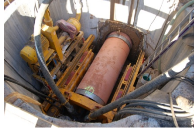
Exit shaft: arrival of the cutting head
