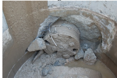
Exit shaft: arrival of the cutting head
