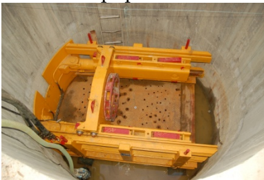
Emplacement of pipe section
