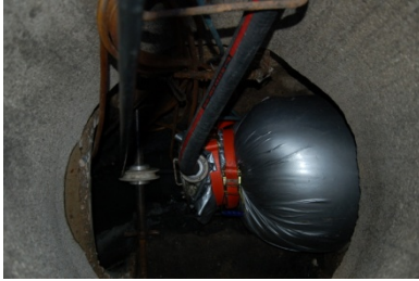
Pipe in curing process
