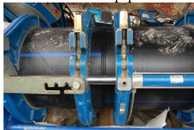
Execution of the weld between pipe
