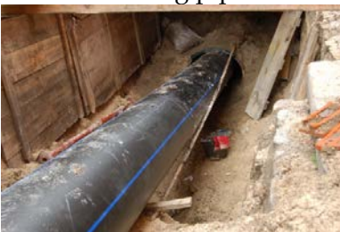
Introduction of lining pipe into existing pipe
