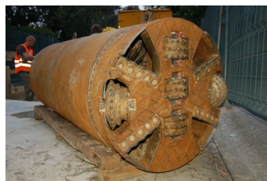
Start to push the pipe section
