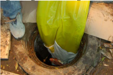
Beginning of inserting of sleeve
