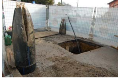
Pulling head and access pit
