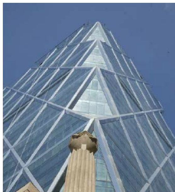
Figura 52: “Bocas de pájaro”. Fuente: Rahimian, A., Eilon, Y. (2008) “Hearst Headquarters: Innovation and Heritage in Harmony.” CTBUG 8th World Congress.
