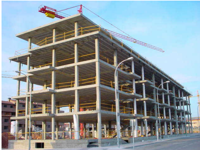
Figure 84: Construction of typical wide-beam frame in Spain
