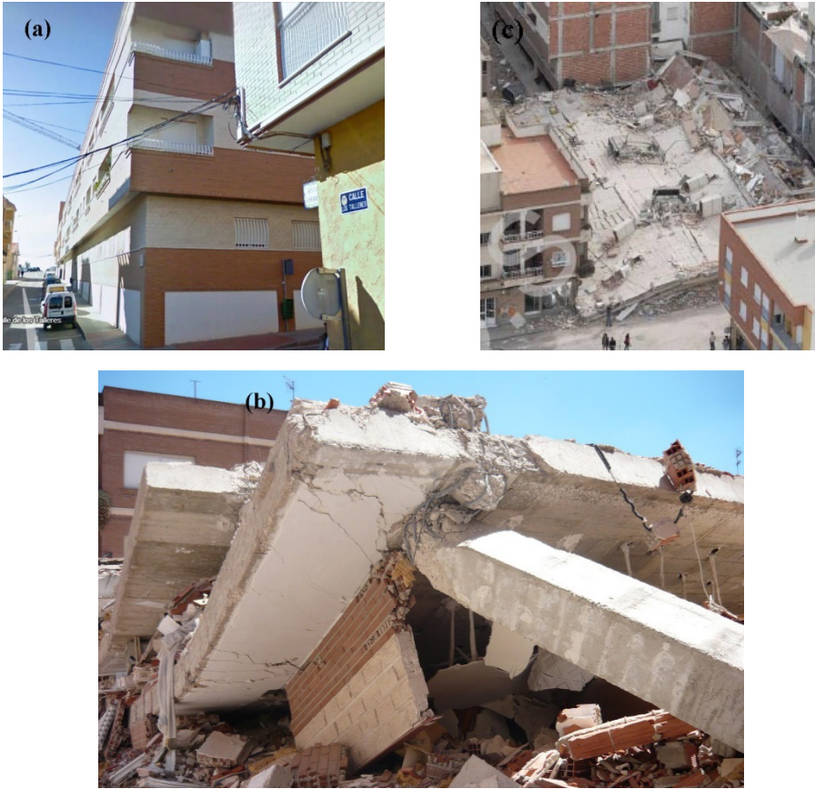
Figure 168: The only building collapsed due to the Lorca earthquake, before (a, from Google Street View) and after the event (b and c)
