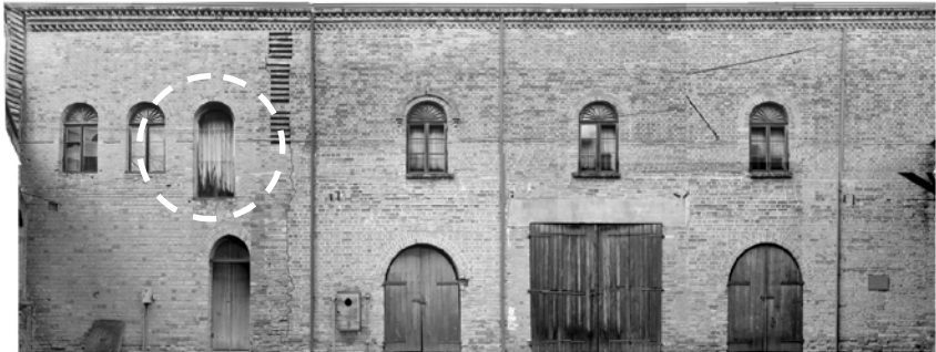
Figure 4. The North Façade of the Lidgerwood M.Co. building: different types of finishing joints that indicate the forecast of expanding the building (G-COR Architecture)
