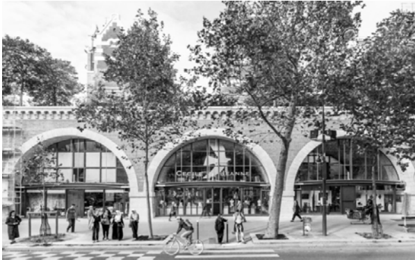
Figure 2. Viaduct of Arts
