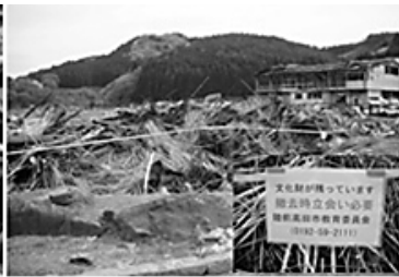
Photo 2. Wreckages of Damaged roof
