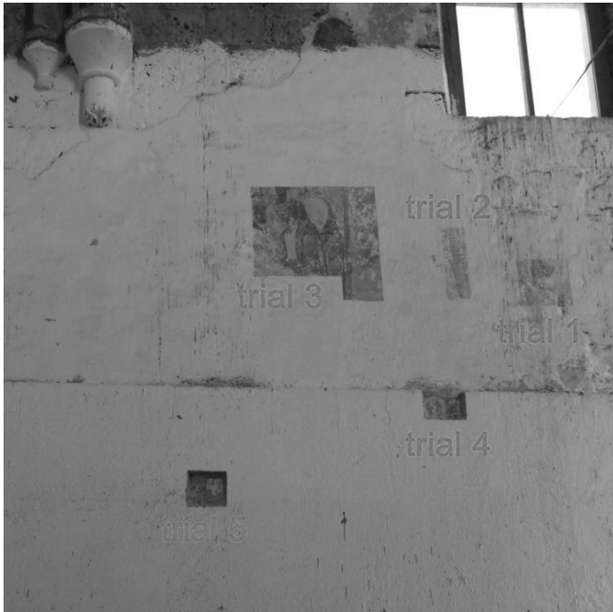
Figure 3. Location of uncovering trials on the south wall
