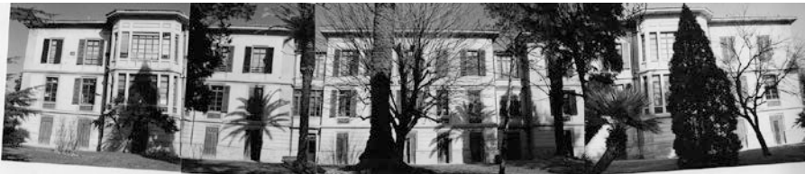
Figure 3 The Villa Ognissanti before refurbishment
