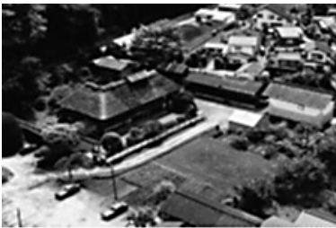
Photo 1. Yoshida's house in 1971.
