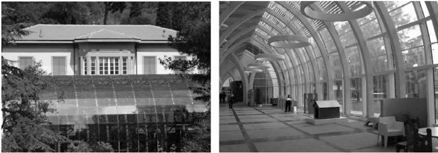
Figure 4 The PV greenhouse
