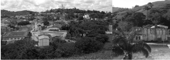
Fig. 6 IPHAN destructive intervention: a shed built on the ruins of Teatro São Pedro , Laranjeiras, Brazil. Photos by Isadora Santana, 2014
