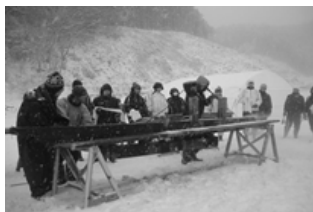
Photo3. To clean the building pieces by engine high pressure water gun
