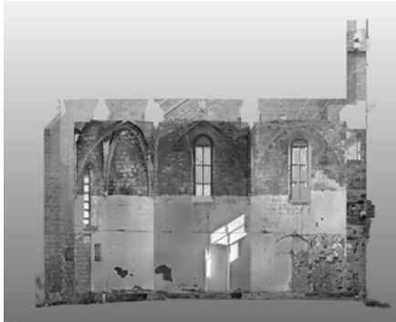
Figure 1: Orthoimage of St. Anne's created from 3D laser scan data
