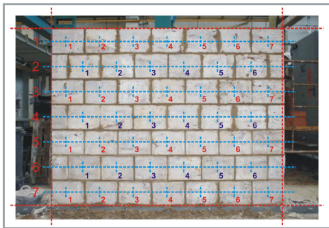
■ Figure 2. Photography of ashlar wall (Wall 2)
