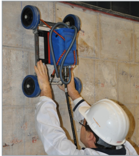
■ Figure 10. Realization of GPR measurement
