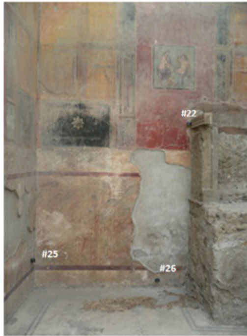
Figure 4.12: Mural frescoes in Ariadne's house (western wall of room 1). Three probes can be observed: #22, #25 and #26, which remain at 240, 54 and 15 cm from the floor, respectively.
