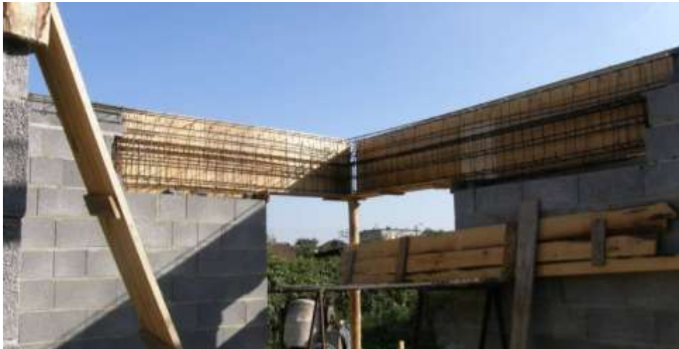
Figure 66 – Lintel connected to the beam. [36]
