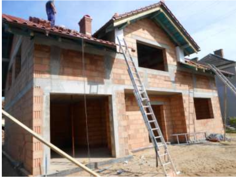
Figure 65 – Lintels above the openings. [35]
