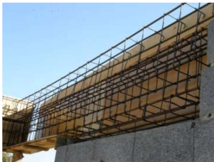
Figure 67 – Lintel connected to the beam. [36]
