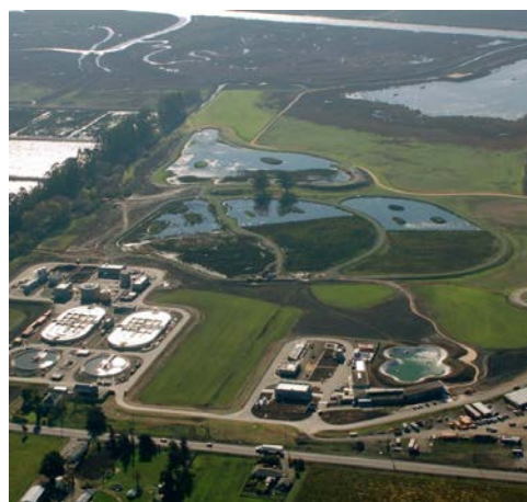
Figura 185. Ellis Creek Water Recycling Facility (2001)
