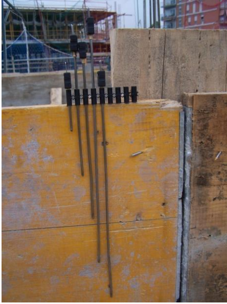
Fig. 4 Thermocouples embedded in floor slab (Sabadell).
