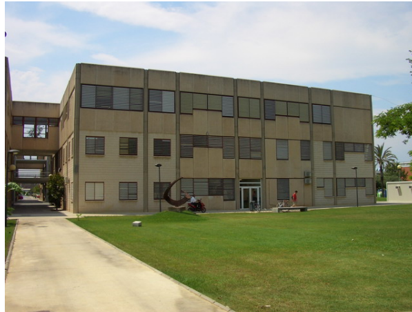
Figure 2.9: Office building of Universidad Politécnica Valencia.
