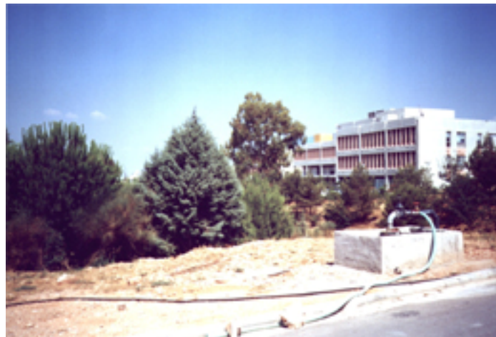
Figure 2.12: Office building of National Technical University of Athens (CRES).
