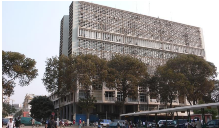
2. Mutamba building – Ministry for Public Works, Luanda (1968) - Vasco Vieira da Costa. (Ana Magalhães, 2008)
