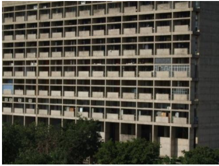
10. The Brise Soleil in The Secretariat, Chandigarh.
