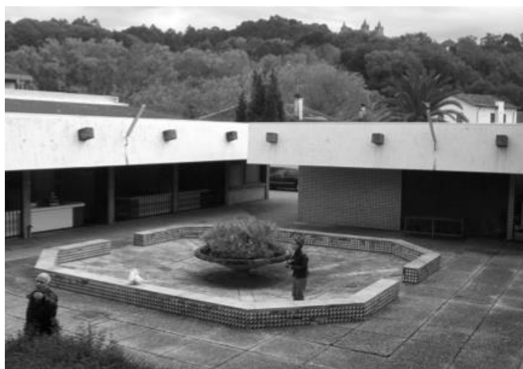
10. Market at Vila da Feira, Portugal. Centre view.
