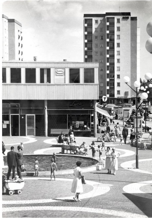
8. Vällingby Centre was designed by Leif Reinius (1907-1995) and Sven Backström (1903-1992)
