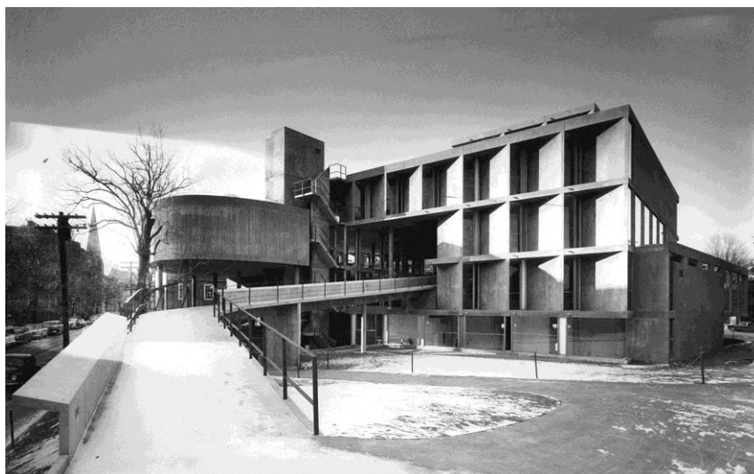
1. Le Corbusier, Visual Arts Centre, view from Prescott Street. © Fondation Le Corbusier-ADAGP, 2015.
