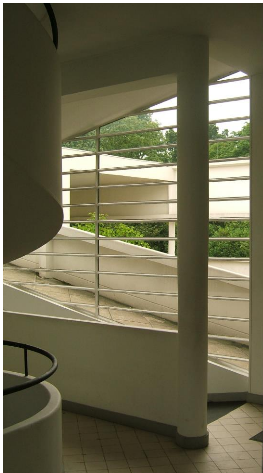
9. Villa Savoye: ramp and stairs (photo Christoph Schnoor)
