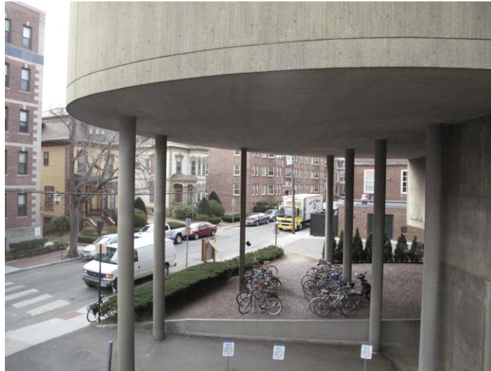
7. Le Corbusier, Visual Arts Center, View under studio space along Prescott Street (© Fondation Le Corbusier-ADAGP, 2015; Camille Tokerud Photography Inc, 2015).
