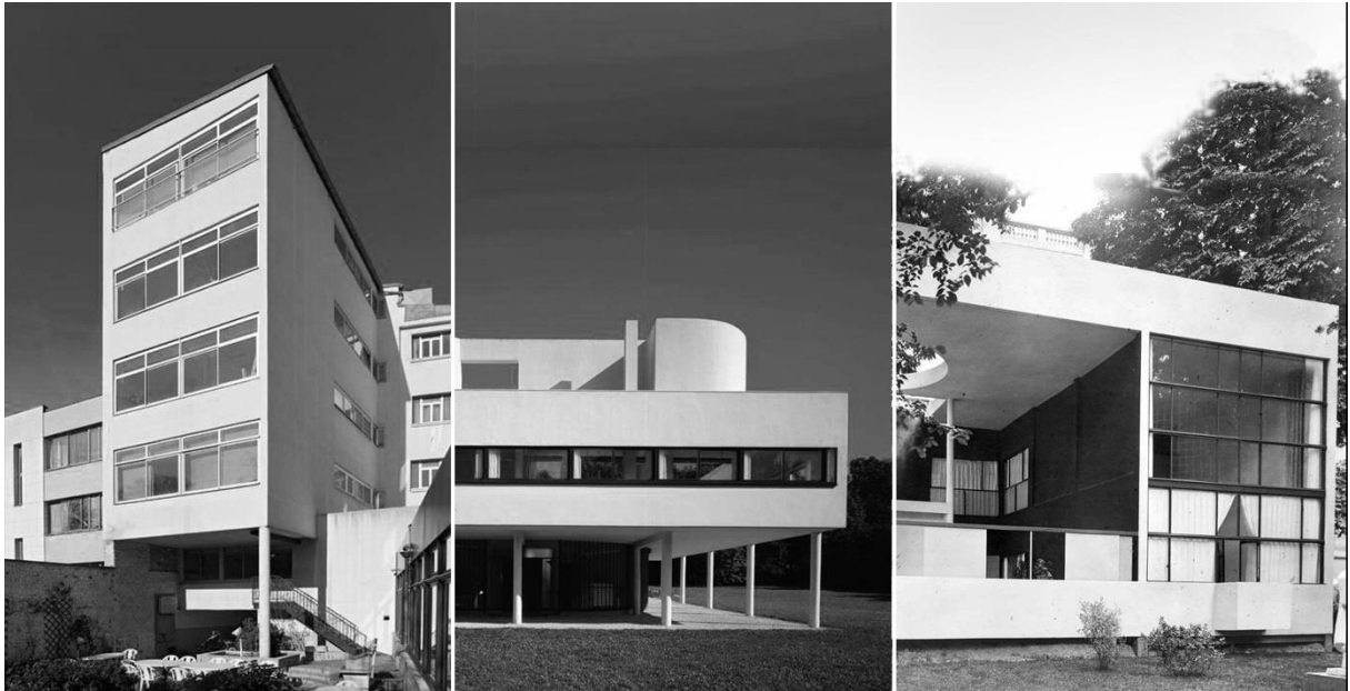
2. Three types of buildings compose the Modern Style of the “Heroic Period” of Le Corbusier in the 1920’s: Residential Blocks, Villas and Pavilions.
