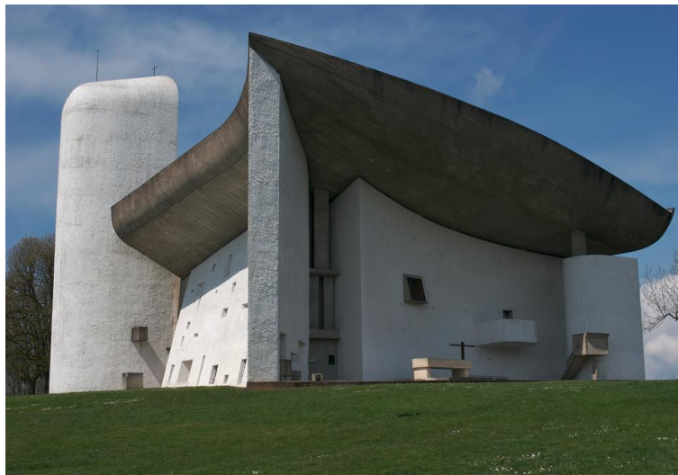
1. Chapel of Notre Dame du Haut, Ronchamp, France, Le Corbusier, 1950. In the east wall there is the open-air chapel.
