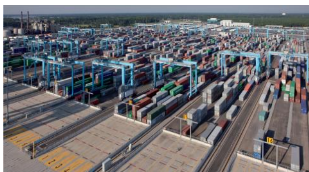
Figura 25 RMGs automáticos (ASCs), APM Terminals Virginia (Port of Virginia - EE.UU.)
