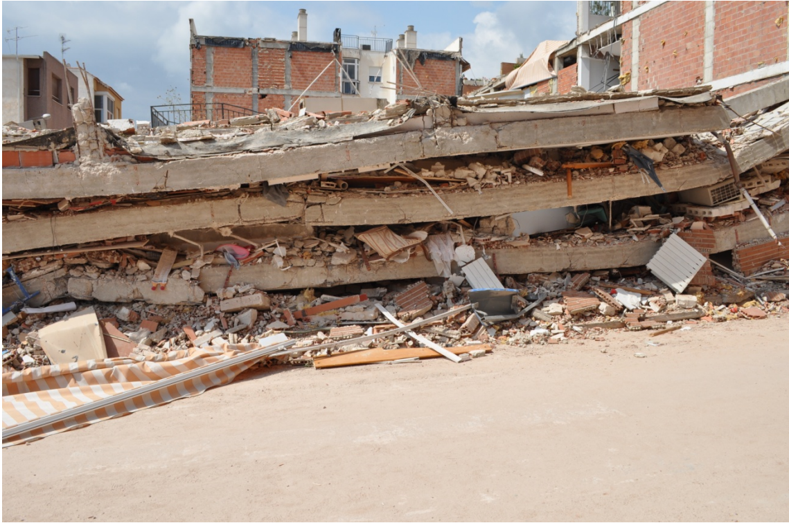
Collapse of a building in Lorca (Spain) during an earthquake in 2011.
