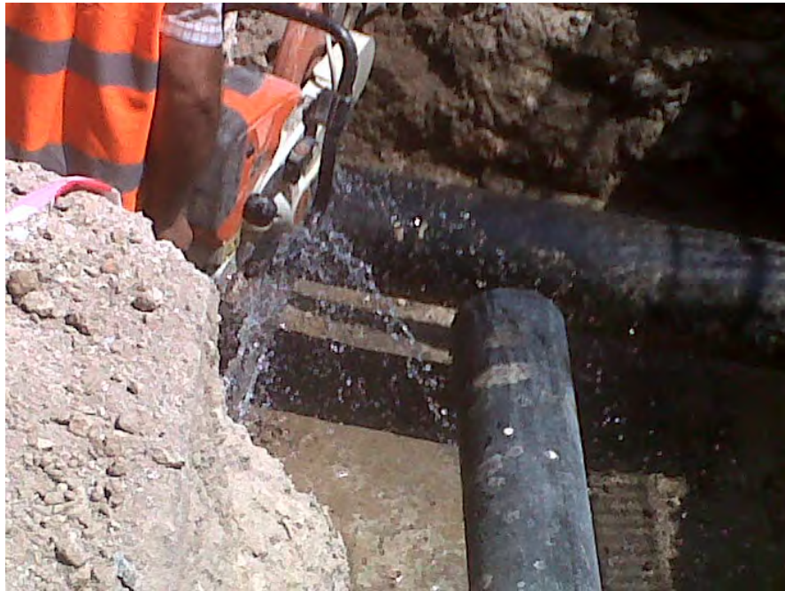
FIGURE 3.7: In situ biofilm sampling in DWDSs. Eva Ramos Martínez ©.
