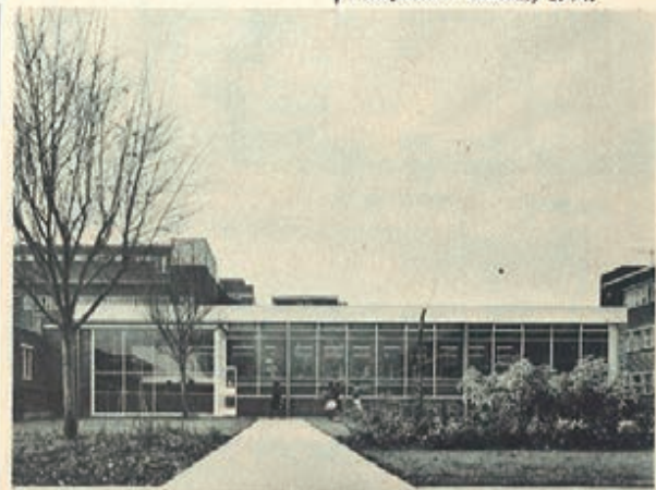
Luton and Dunstable dining room servery and coffee lounge Completed – February 1974.
