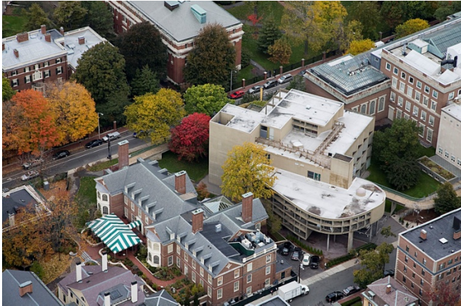
Carpenter Center for the visual arts, Boston, 1959-1963
