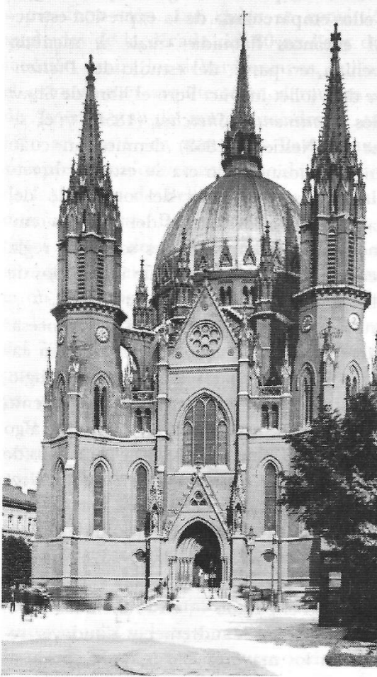
A Fachada Principal
