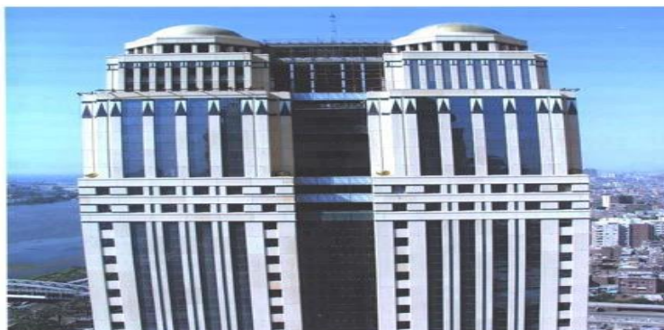
Figura 23 Nile City project, Egypt. 2 x twin Towers (Mármol Salazar, 2010)
