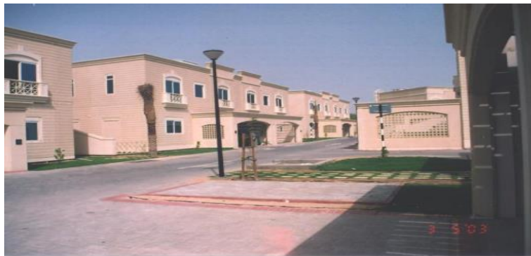
Figura 21 GFRC Insulated Wall Panels for Modular Housing in Dubai (Mármol Salazar, 2010)
