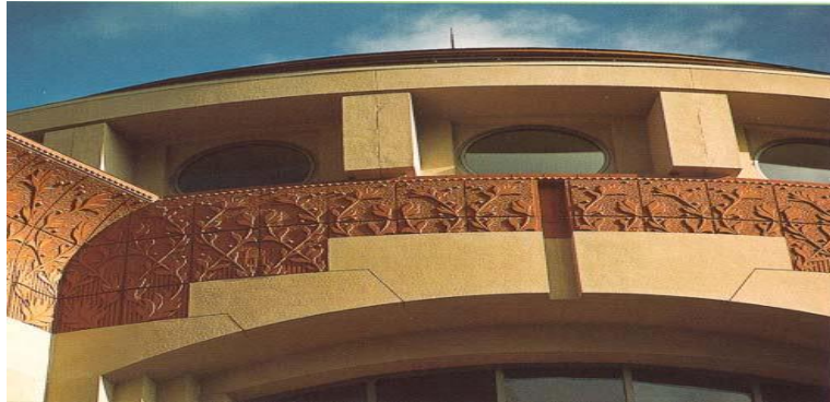
Figura 22 GFR panels on the Cervantes Convention Centre, StLouis. 2 finishes Ornate/pigmented and stone simulation (Mármol Salazar, 2010)
