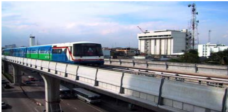
Figura 24 Bridge Parapets, Thailand (Mármol Salazar, 2010)
