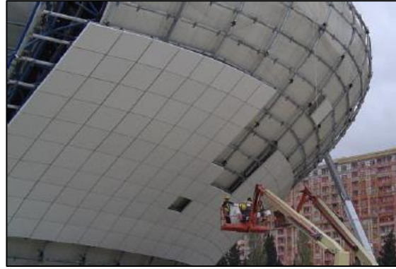
Fig. 2. Double-curved cladding elements: Heydar Aliyev Cultural Centre (Baku, Azerbaijan)
