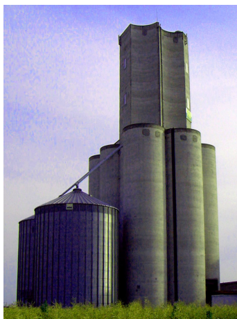
d) Older concrete and newer steel silos, France
