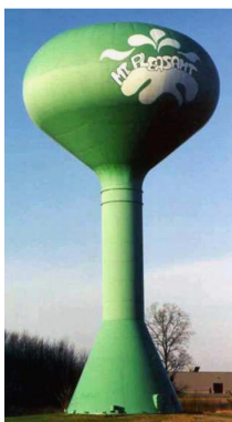
b) Elevated water tank, USA
