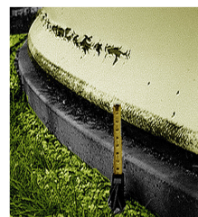
d) Elephant's foot: seismic action
