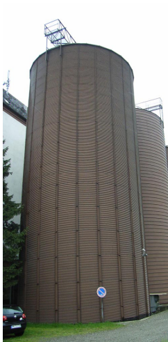
b) Corrugated steel storage, Germany
