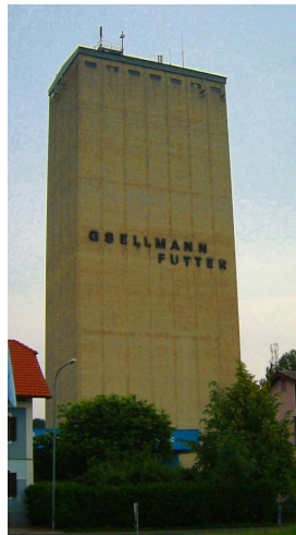
c) Rectangular concrete silo battery, Austria
