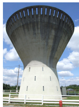
c) Concrete elevated water tank, France
