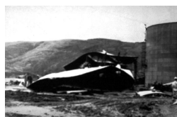
c) Tank separation from foundation, USA
