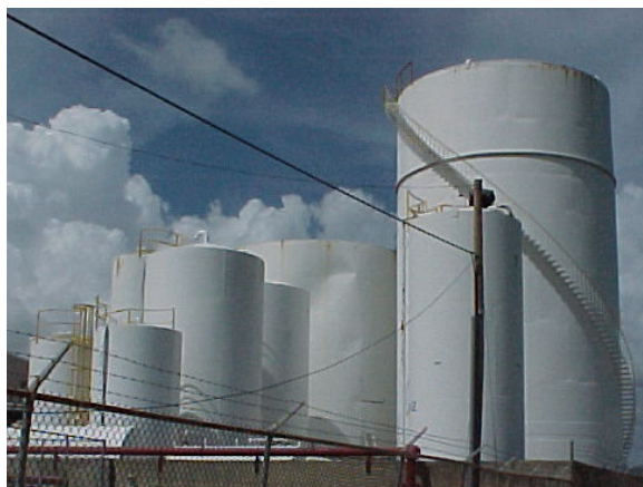
Figure 1. Group of tanks in a tank farm, showing buckling of the central tank following Hurricane Georges in Yabucoa, Puerto Rico. (Photograph by the author)
