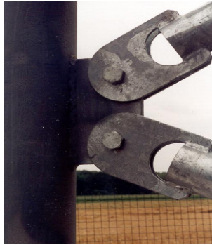
Figure 6: Traditional joint between diagonal and legs, both circular tubes. Austria
