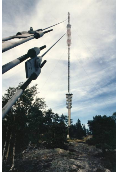
Figure 9: The parabolics are fixed to the stiff concrete tower
