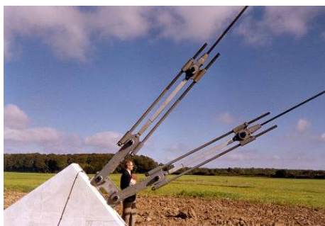
Figure 11: Guy attachment to foundation with tension system
