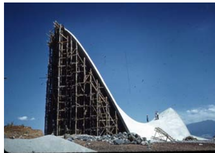
Figure 7: Chapel Lomas de Cuernavaca, 1958, under construction.
