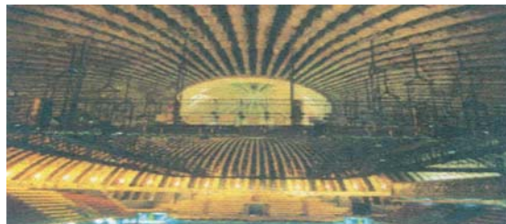
Figure 2(b): Example of precast folded plate dome
