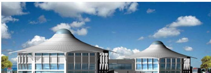
Figure 1(a): Example of cast-in-place shell
