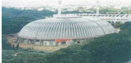
Figure 2(a): A dome of 90m x120m using precast folded plate elements
