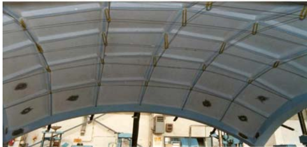
Figure 9: Elliptic shell prestressed by inside
