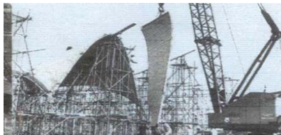
Figure 4: Precast elements being placed in position
