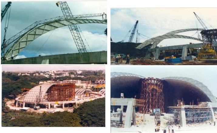
Figure 7: Erection process of precast elements
