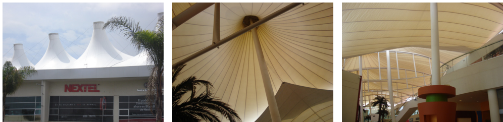
Figures 13, 14, 15: Exterior and interior views of Palmas Plaza (photos: J. Mundo, 2008).
