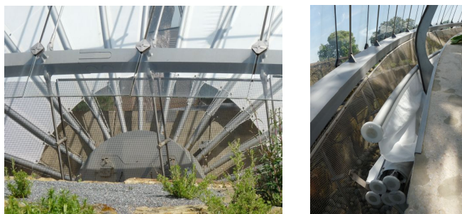
Figure 22: Deployable screens shade the interior of the Alpine House (photos: R. Baker).
