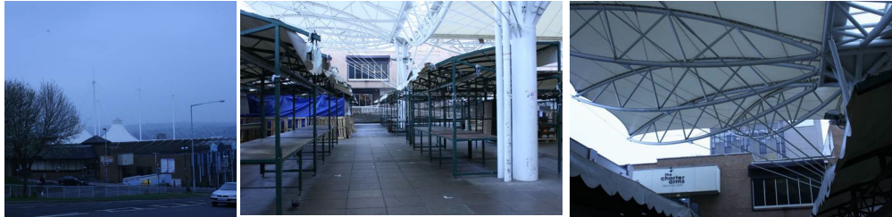
Figure 16 (left): Exterior view of Rotherham Market (Photo: Architen Landrell). Figure 17 (centre): Free standing masts (Photo: M. Mendoza, 2009). Figure 18 (right): Flanking membrane elements flying over the existing building (Photo: M. Mendoza, 2009).
