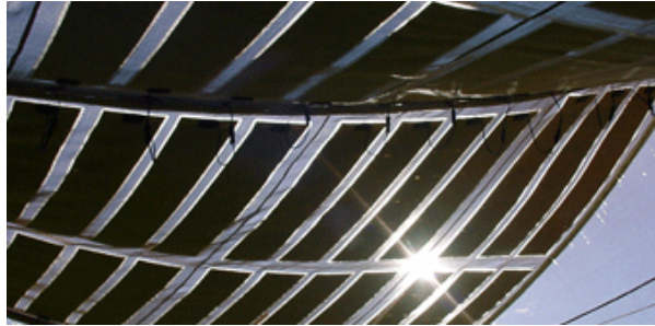
Figure 23: Thin film solar cell embedded onto a roofing membrane.
