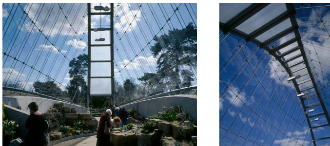
Figure 21: Height contributes to the stack effect of the Alpine House (R. Baker, 2009).
