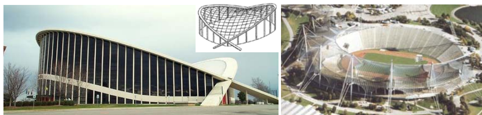
Figure 2: Closed Cable Mesh: Raleigh Arena (USA, 1953); Open Cable Mesh: Munich Olympic Park (Germany (1972)).
