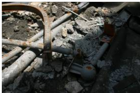
Figure 4-k: (↑) members and nodes fell down on the ground (1) Figure 4-m: (→) members and nodes fell down on the ground (2)
