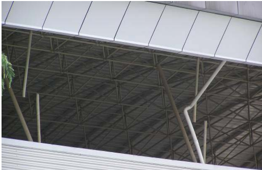
Figure 2-c: (↑) member failed under tension forces
