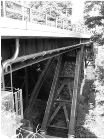
Photo 2 : The Bridge to which T-BRB is applied
