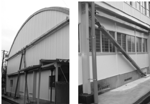
Photo 3 : The gymnasium after reinforcement
