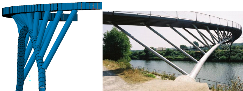
Figure 10: (Left) Example of spatial arch bridge composed of an antifunicular arch and an upper deck (Right) Ripshorst Footbridge, by J. Schlaich.
