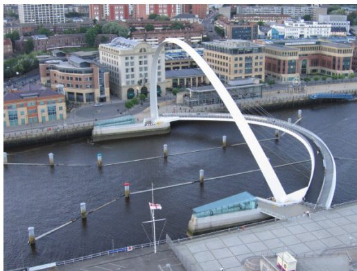
Figure 4: Gateshead Footbridge (Johnson and Curran [1]).
