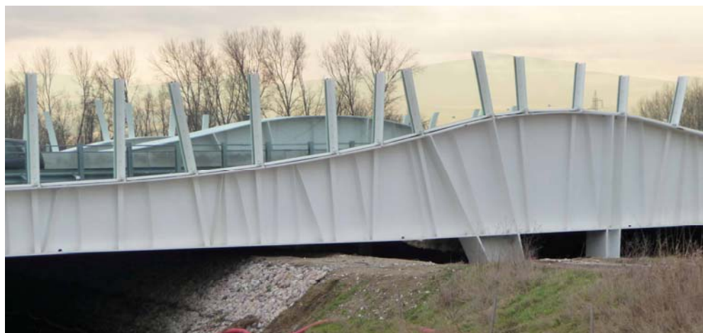
Figure 4: The bridge under-costruction
