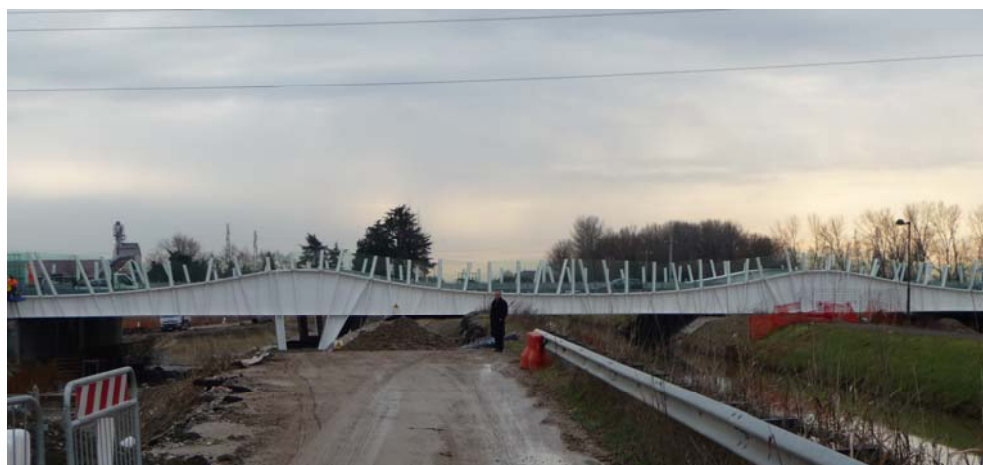
Figure 5: The bridge under-costruction
