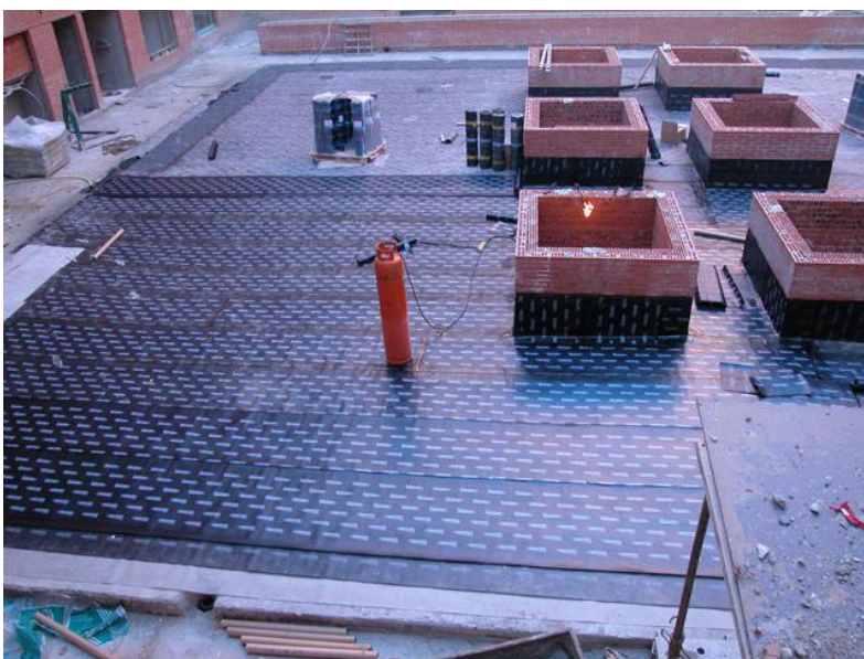
Figure 32. Waterproofing
