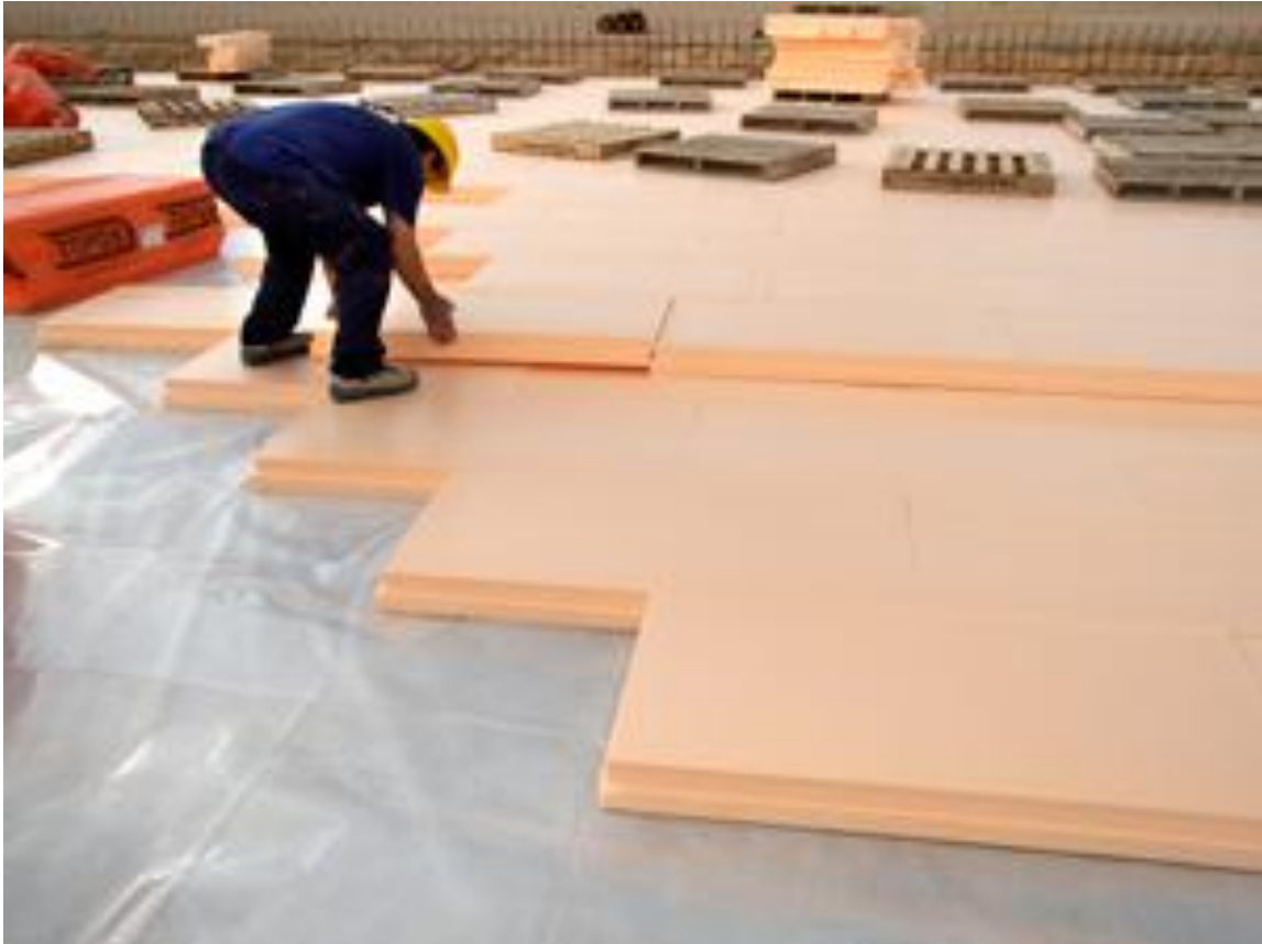
Figure 31. Thermal and sound insulation
