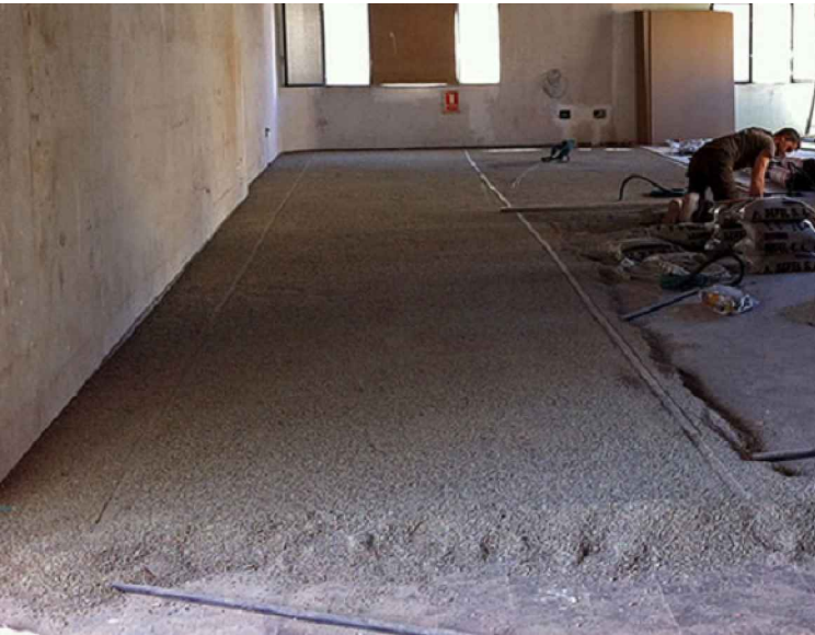
Leveling with sand layer
