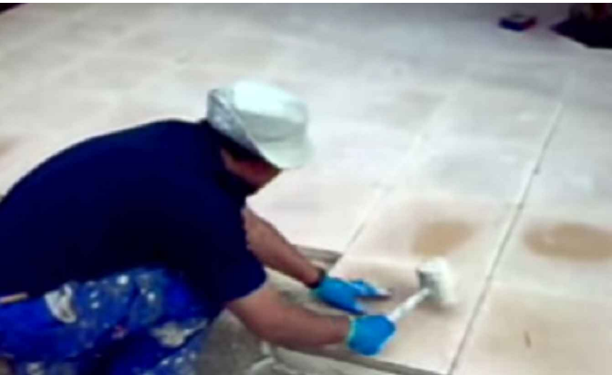
Fix and level with rubber mallet
