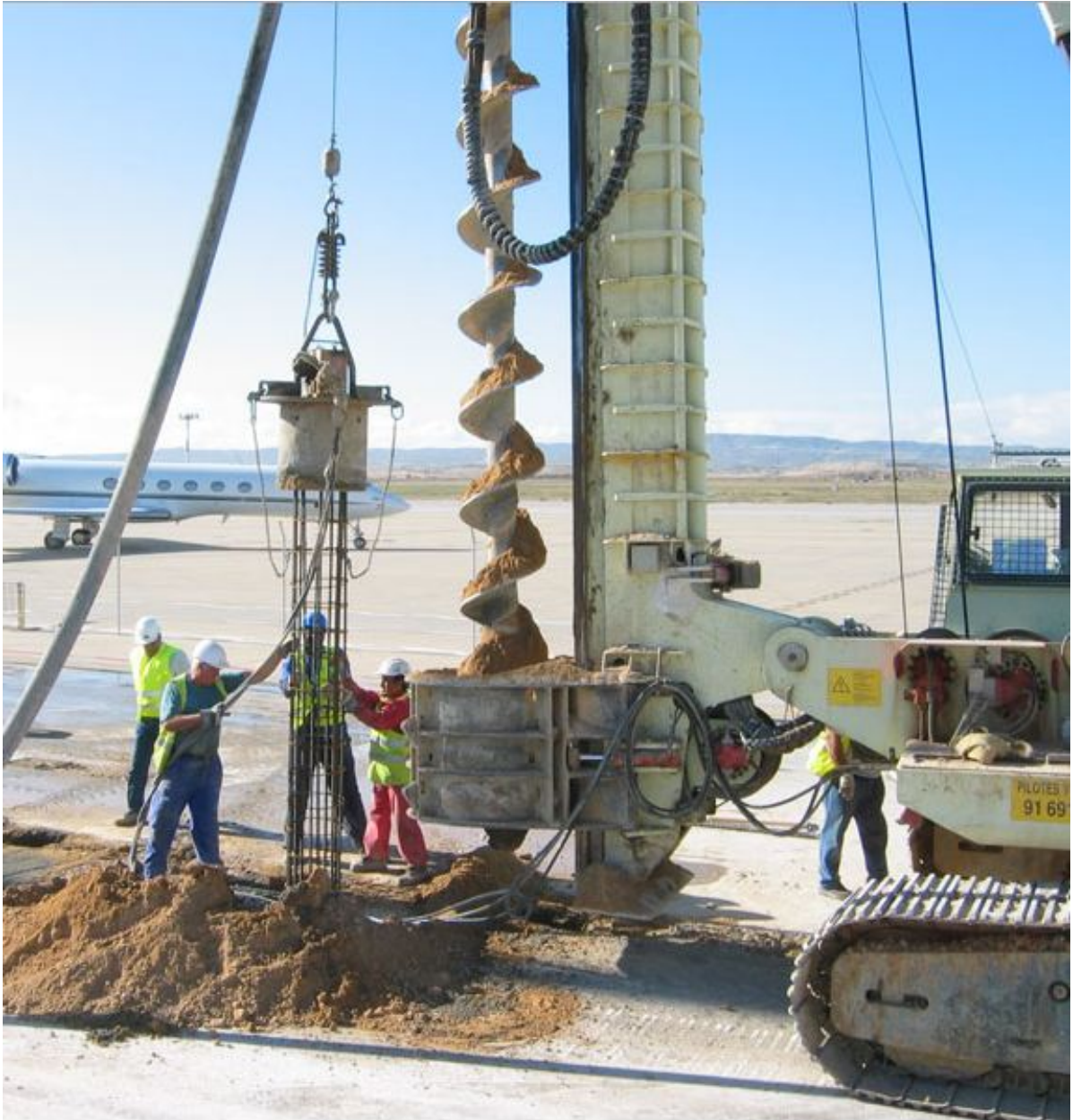
IMAGE 3 . Continuous flight auger equipment
