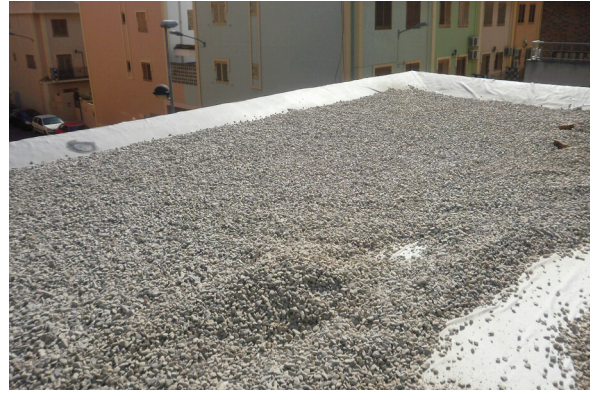
Image 7 and 8 . Placement of insulation layer and gravel.
