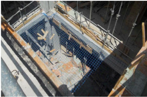
Image 9. Horizontal red to protect the holes.
