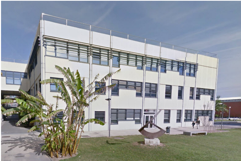
Figure 2.2: Department of Applied Thermodynamics building.
