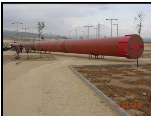
Fig. 4. Photography of the complete-assembly before holding monopost up.
