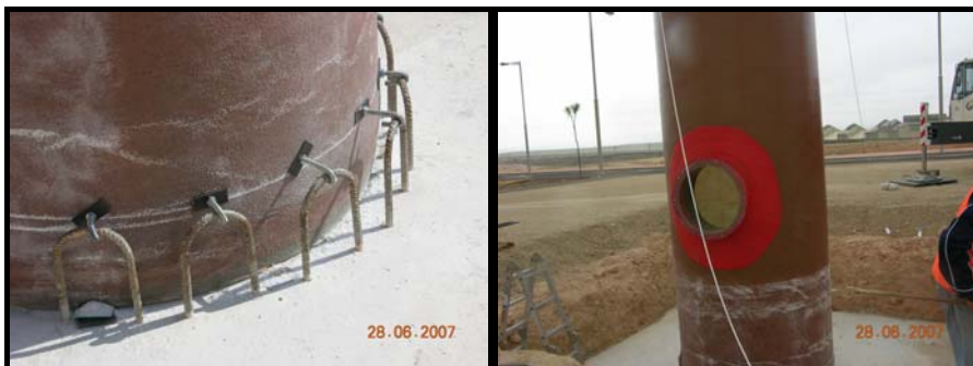
Fig. 10. Photographs of anchorage system: forks, screw bolts and monopost.
