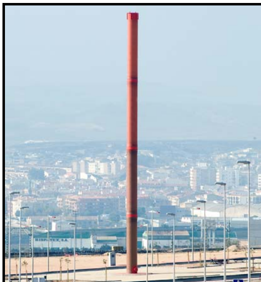
Fig. 2. Photograph of day view of monopost and surrounding area.
