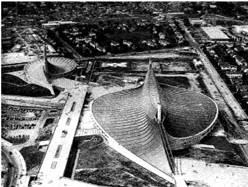
Figure 5: Tokyo Olympic Swimming Pool, 1967 of Tsuboi & Kawaguchi (Irvine).
