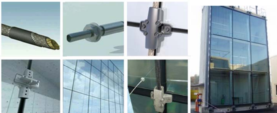
Figure 6: Walls examples and some details realized by GIG. PBO Cables, Austria (Future Fibres Company).
