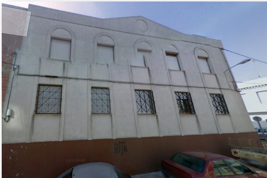
Figura 4. Fachada principal .2013. Google Maps.
