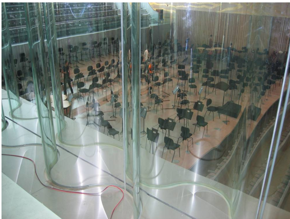
Fig. 3. In between the two corrugated glass walls a cavity to reduce the sound level between the two spaces.
